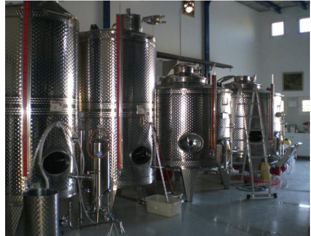
©Zambartas The modern winery installation
